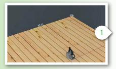
Put shower tray in the correct position and mark around the tray, to establish which section of the floor boards need to be removed, the tray can be recessed.
