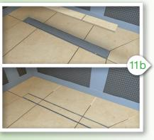
If you're using a tile on grate, the height of the stainless steel support can be adjusted utilising the height adjustment spacers, but the inner height of the tile on the grate is fixed (13mm). Please ensure that you use suitable tiles for the grate and the shower tray.
